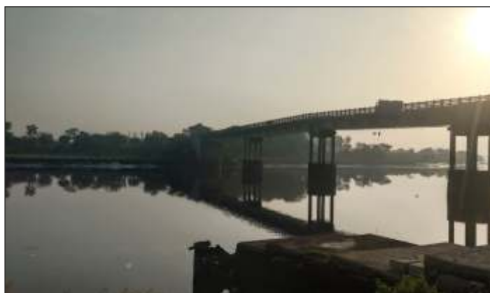
Fig. 5: Survey area of Ulhas River, Gandhari Bridge
