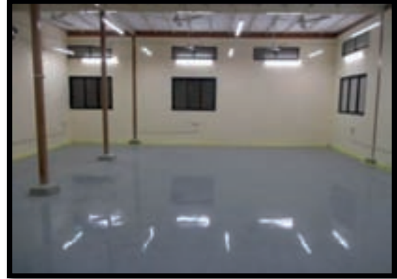
Radiography Device Maintenance Shop-floor at Integrated Facility for the Industrial Radiography Device (IFIR)
