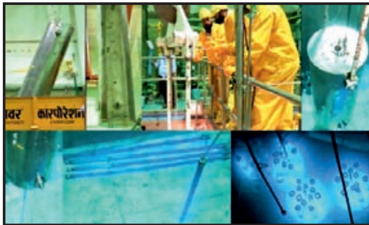
Fig. 24: Discharging operation of highly radioactive Cobalt-60 Adjuster rods received from RAPS Unit #4 in RAPPCOF Storage pool
