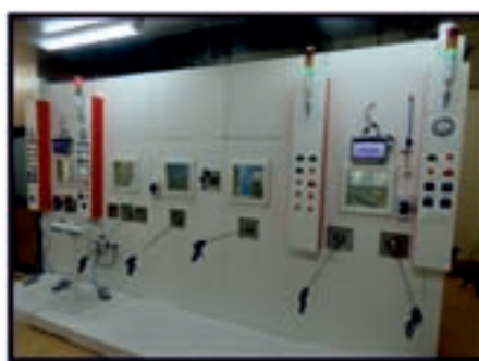
Fig. 11: Hot commissioning of new advance facility for production of ^{131}\text{I} capsules in RPL
